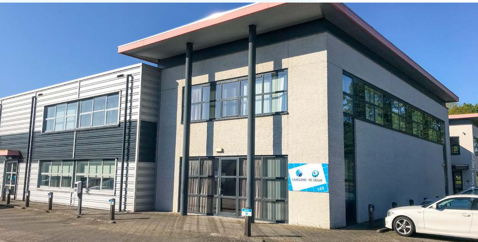
LAAGLAND is a long-time distribution partner of MAPAL's. The company's headquarters is in Capelle aan den IJssel near Rotterdam.
